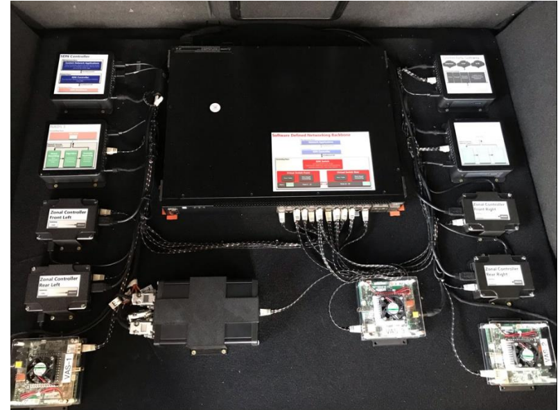
Installation in the trunk
