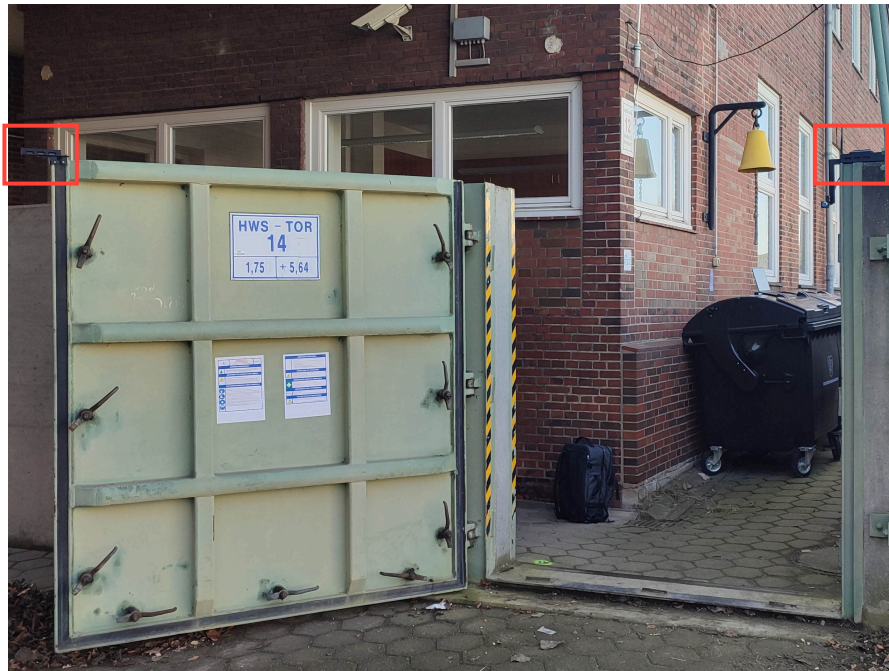
Figure 13: Full view of the open floodgate with the mounted housings on the gate and the frame.
